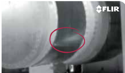
Captured gas leak from production site.
