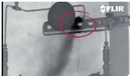
A leaking LPG treater.
