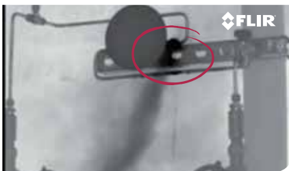
A leaking LPG treater.
