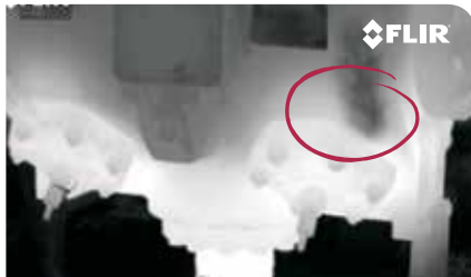
Captured gas leak.
