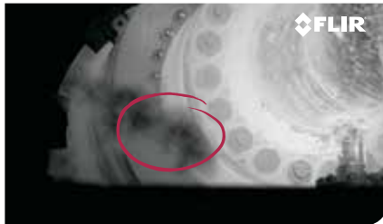
A leaking flange.
