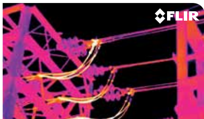
Continuous monitoring of a high-voltage installation.
